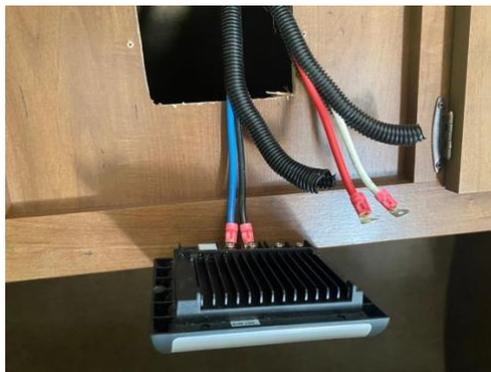
*Figure 7: Wires should be spliced blue to red and white to black*
