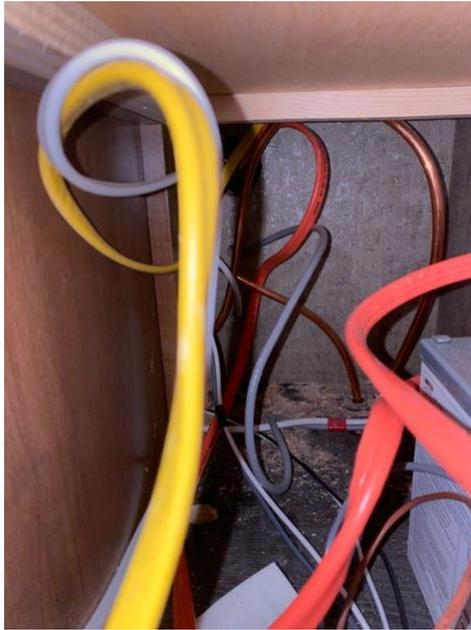
*Figure 10: Propane lines penetrating trailer floor at the back of the picture*
