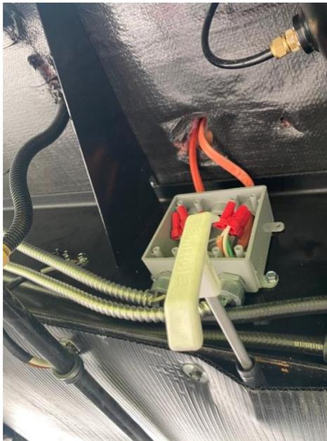
*Figure 13: Two splices; one to transfer switch and one to distribution panel*
